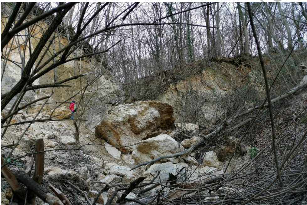
Figure 16. Coseismic slope failures caused by the 2020 Petrinja earthquake sequence. Top) The landfill landslide of the Međurače quarry (Paleogene rocks) (ID 434; latitude 45.432899, longitude 16.179700). Bottom) Rockfall located within the fault zone in highly fractured Badenian calcarenites at the head of a gully. West of Hrastovica (ID 170/ latitude 45.3972938, longitude 16.2815195).
