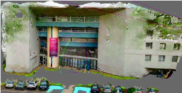
Figure 5: 3D reconstruction of the main building from the overlapping views using Structure-from-Motion [1].
