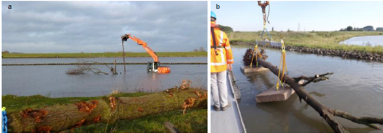
Figure 2: a) Trees are placed in shallow zones along the river b) Trees weighted with concrete slabs are placed in erosion pits behind groynes, up to 9 meters deep.
