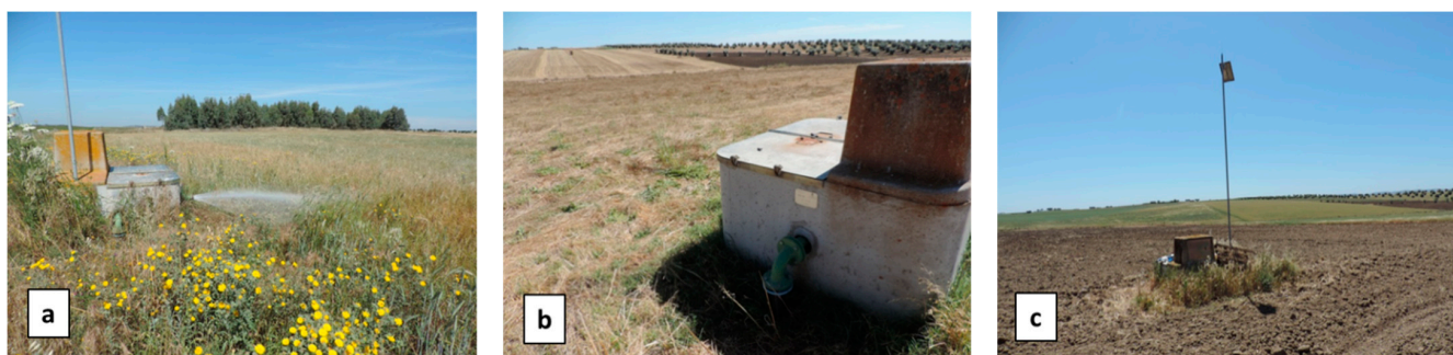
Figure 11. Pictures in May 2019 of (a) hydrant H5.6, (b) hydrant H10, (c) hydrant H11 and the corresponding environment, respectively, a meadow with high grass, a meadow with short dry grass, and bare soil. The picture in (a) was taken while the valve was open to simulate a leak.
