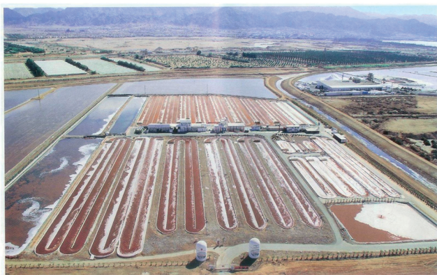
Fig. 5 Raceway of 3000 m 2 in NBT, Israël ( https://www.israel21c.org/wp-content/uploads/2016/02/algae-NBT.jpg ) 65 (this figure was published in P. J. Harvey and A. Ben-Amotz, Algal Research , 2020, 50, 102002, Copyright Elsevier).
