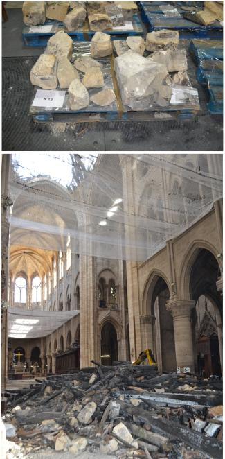
Figure 1: Examples of pictures taken in the context of a restoration site. Top: A pallet of debris (Claudine Loisel / LRMH) Bottom: The debris in the nave of the Notre-Dame cathedral (Aurélia Azéma / LRMH)
