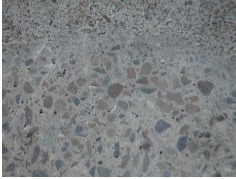
Figure 1: Surface of concrete showing multiple aggregates (image from wikipedia.org).
