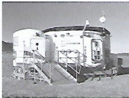
Habitat Demonstration Unit Pressurized Excursion Module (HDU 1-PEM) is a one-storey, three-port habitat unit. Engineers are evaluating the habitat design concept during the 2010 field tests. Image credit: NASA.
