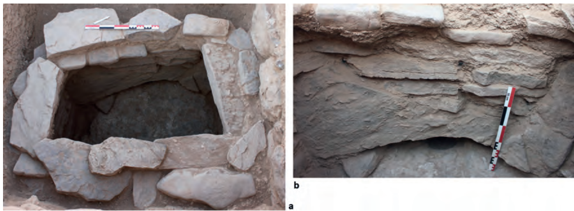
Fig. 4 'Cistern' 3066: a. view from the west; b. detail of the east wall (M. Jean/FAMCO)
