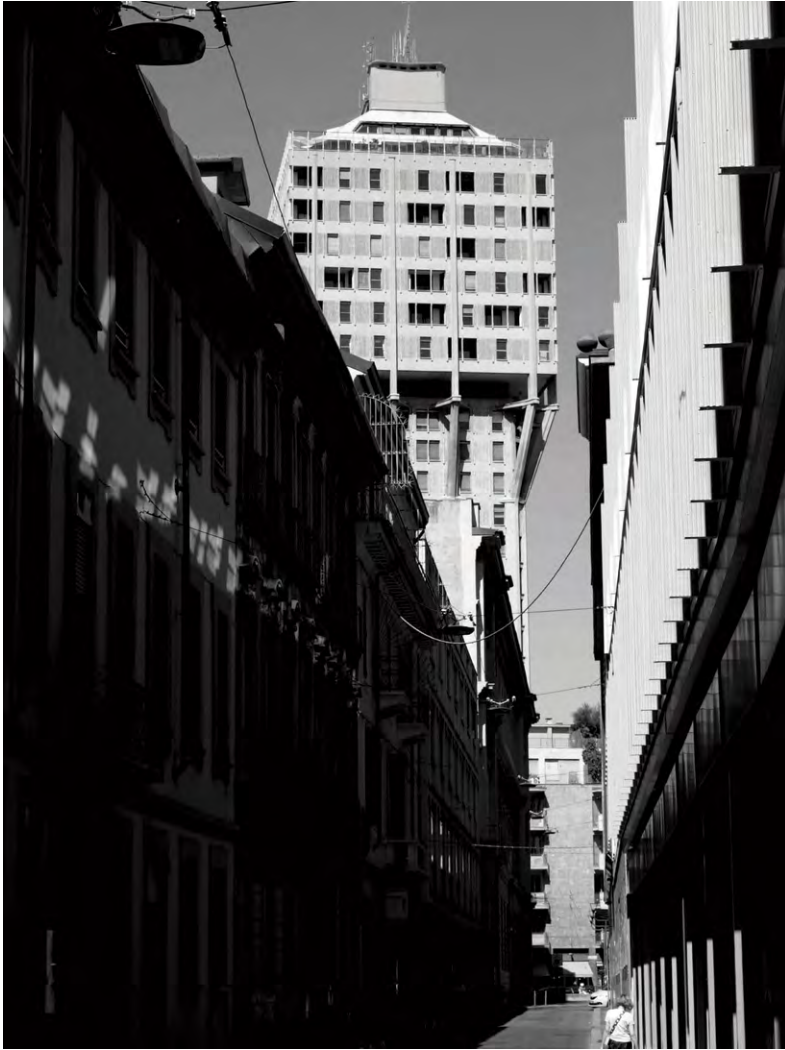
Figure 5.2 BBPR, Torre Velasca, Milan, 1956–8
