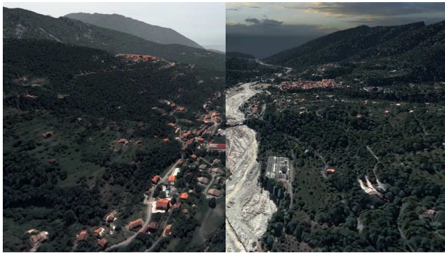
Fig. 4. QUB 3D multi temporal scene – Split view of 2019 & 2020 Vésubie valley (flood damages on the right picture)
