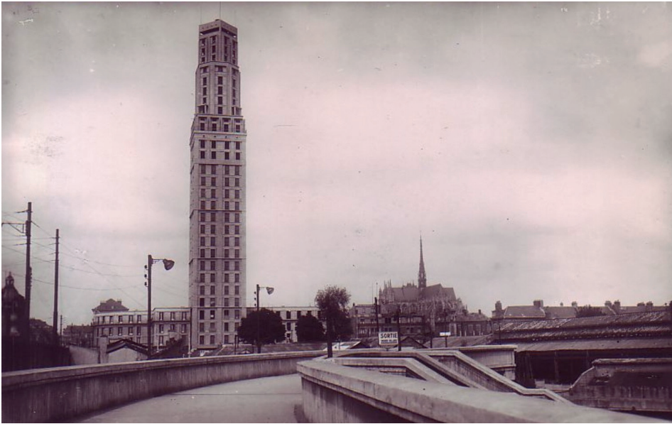
◀ Fig. 5. The concrete carcass of the Perret Tower from the station, postcard, 1950s (© DR).
