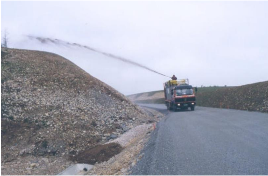
Figure 1. Utilizing hydroseeding technique as a restoration tool on a steep road cut slope.
