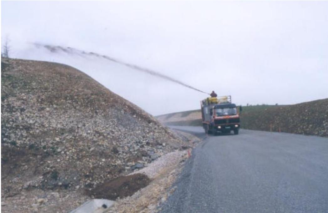
**Figure 1. Utilizing hydroseeding technique as a restoration tool on a steep road cut slope.**
