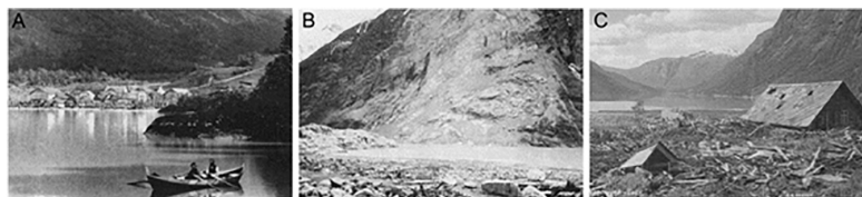
FIGURE 2 | (A) The settlement of Bødal in CE 1890. (B) The Mt. Ramnefjell slide scar following the 1936 rock fall, with remains of Bødal in the foreground. (C) Remains of the settlement Bødal following the rock fall and tsunami event in CE 1936. Following the two events, the settlement was rebuilt 50 m above its past location in order to avoid destruction from a future event. All pictures are from Martinussen and Berg (1937).
