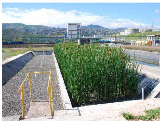
Figure 2: View of the planted and unplanted subsurface-flow wetlands treating the effluent from an UASB reactor.
