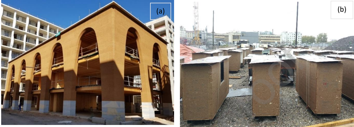
Figure 1 : The case study building with unstabilised rammed earth (RE) with a load bearing façade, in Lyon (France) (a) view from the South-East (b) Picture of the premanufactured RE blocks, contractor: Meunier le pisé, structural engineers: Batiserf, architects C. Vergely Agency (©: Fabrice Fouillet for (a) and Pelé-Peltier for (b))
