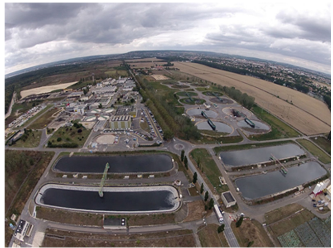
PHOTO 5.2.1 The Seine-Aval wastewater treatment plant, the largest in Europe. Taken in September 2012. https://fr.wikipedia.org/wiki/Station_d%27%C3%A9puration_Seine_Aval . Accessed 25_02_2019.
