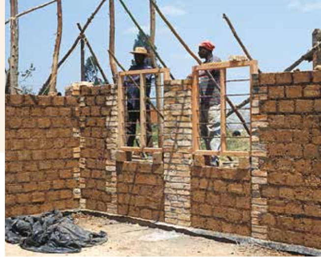
Building site combining different local materials (fired bricks and MEB)
