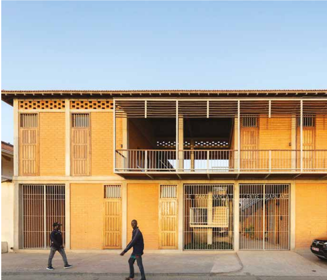
Diapalante Centre, Saint Louis, Senegal Architects: Suzanne Hirchi and Laurent Biot Company: #ELEMENTERRE
