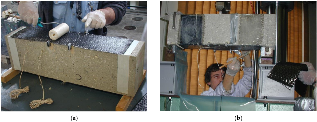
Figure 6. Strengthening of specimens: (a) beam ES1 positioned upside down; (b) CFRP strips bonded as in the field (technicians working under the beam ES2).
