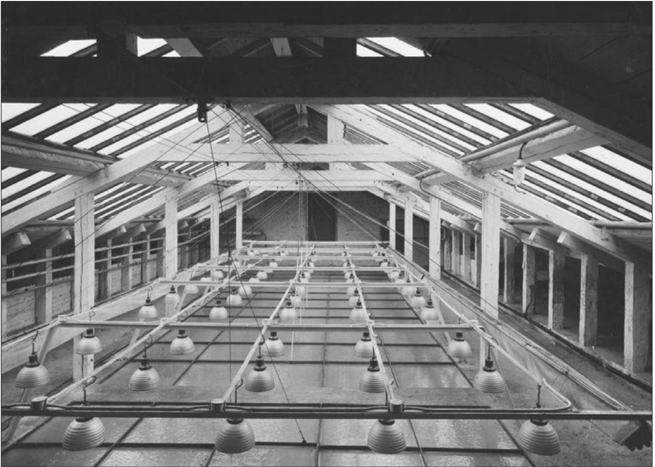
Figure 4 - Nationalmuseum, Stockholm. Lighting installation under the ceiling, second floor, painting room, 1931. Archive number 20/24. Ingenjörsbryån, SFV archive (The National Property Board). (© Nationalmuseum, Stockholm)
