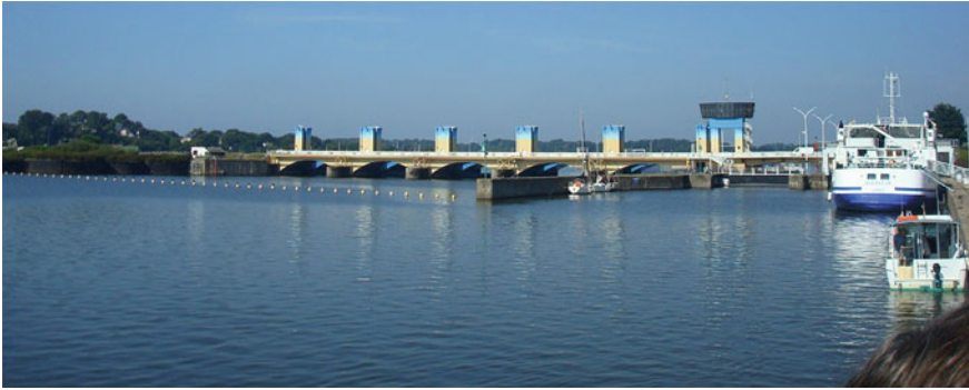
Fig. 6.3 The Arzal dam ( Source IAV, with authorization )
