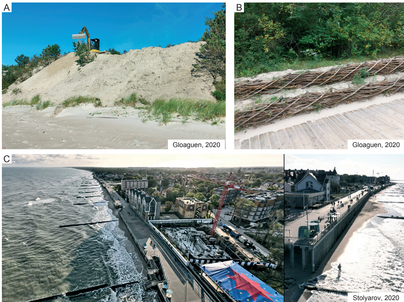
Fig. 7 Coastal protection measures. [A] Beach dune resurfacing and reinforcement works in the Lithuanian mainland coast. [B] Protection of the dune crest by natural materials with special fencing in Palanga. [C] Protective structures in the cities of the Sambian Peninsula, the beach is surmounted by several groynes and overhung by a seafront wall used as a promenade (with Google Street View)
