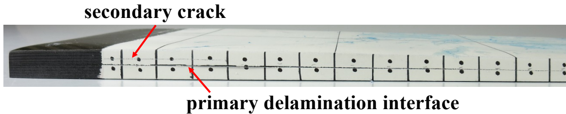
Figure 24: Photograph taken post-impact showing evidence of a large, primary crack close to the mid-plane from test CP5; a small, secondary delamination has also been highlighted
