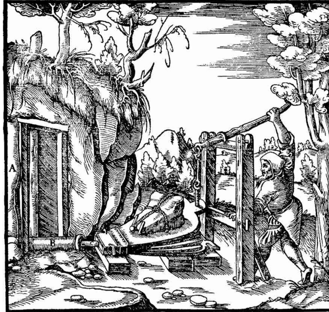
Figure 3: De Re Metallica (1556), book 6, fig. 209. The ventilation system consists of one gear located at the mine's entrance connected to a conduct set on the floor and entering the gallery.
