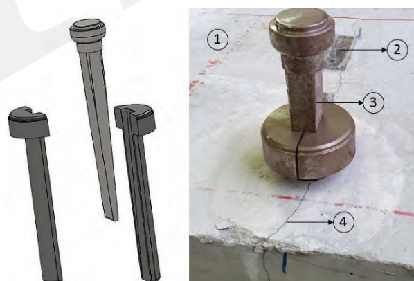
Figure 3. Wedges used for cracking concrete with: (1) lower side of the slab, (2) thin steel plate, (3) wedges and (4) hairline crack.
