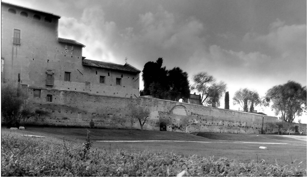
Fig. 3. View of the southern wall, which separated the Heliogabalium from the Domus Augustana (© Ch. Durand, AMU-CNRS, CCJ).
