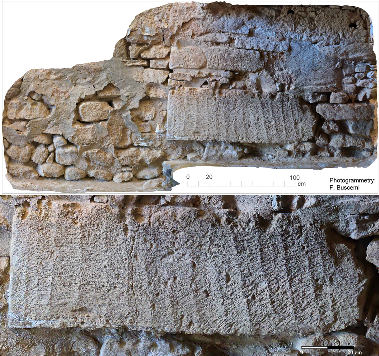
FIG. 9.5 PHAISTOS PALACE. REUSED BLOCK IN THE NORTHERN WALL OF CORRIDOR L, IN CONTEXT AND DETAIL (PHOTOGRAMMETRY BY F. BUSCEMI)
