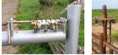
Figure 2: Two ad-hoc physical 1-out-of-6 locks.
