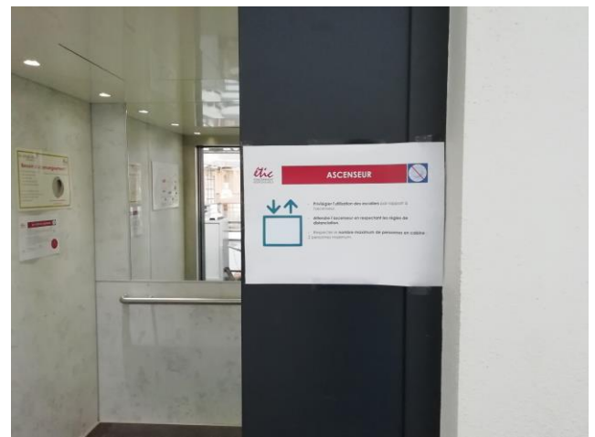
Fig. 10 Restriction to 2 passengers maximum in an elevator which normal limit is about 13 people (1000 Kg). Co-working office ‘Le 22’, Castres, France
