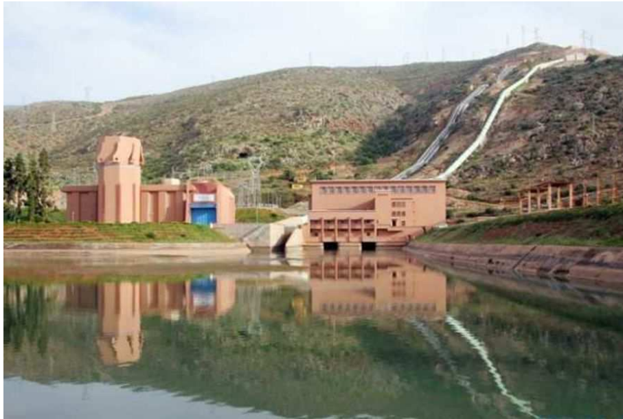
Fig 6 : Hydroelectric Plant near Agadir – Morocco [42]
