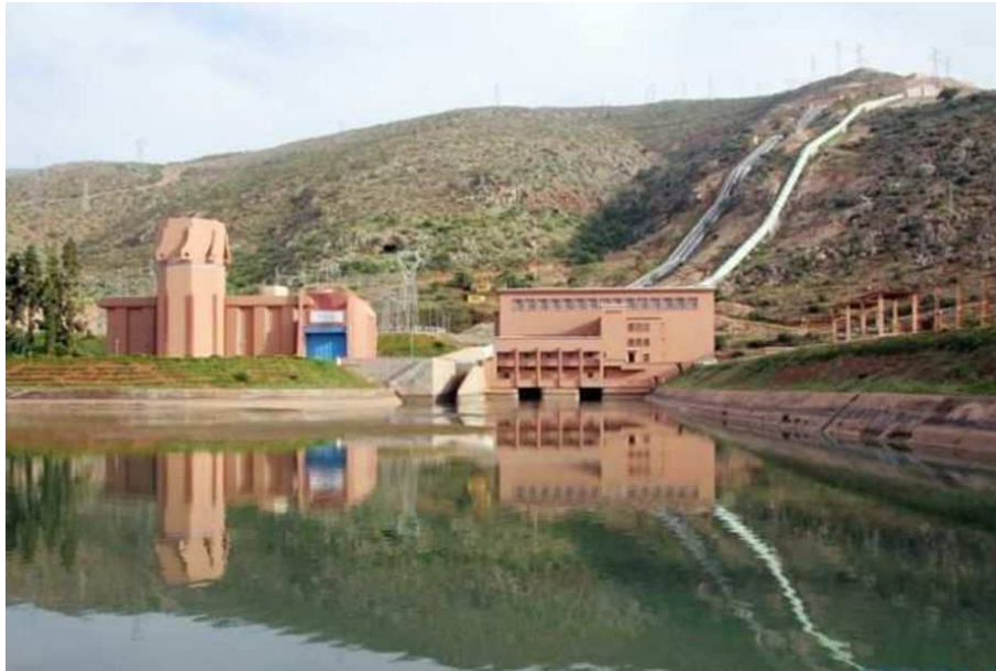
Fig 6 : Hydroelectric Plant near Agadir – Morocco [42]
