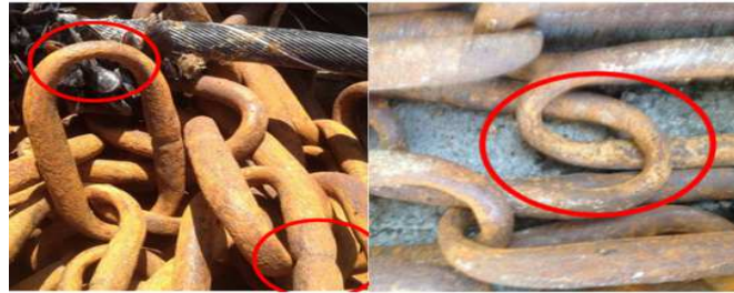
Fig. 3. The corroded chain mooring lines of a meteocean buoy at the SEM-REV sea test site (Berhault, 2017).
