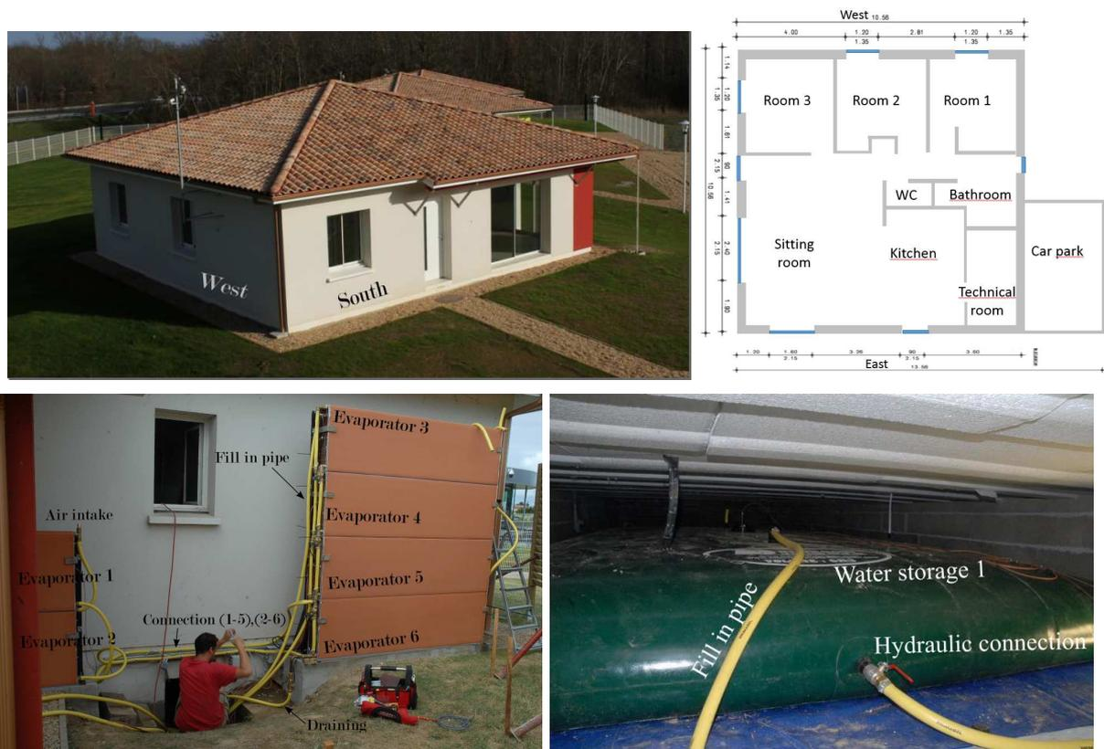
Figure 2: Views of the experimental house, the evaporator and the storage installation
