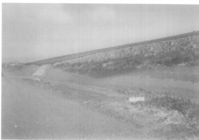
Fig. 3. Filled former large gully of hillside.
