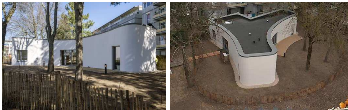
Fig. 6 a) The finished social housing.
