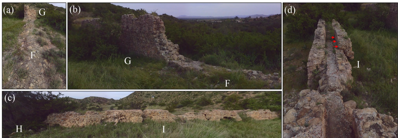
Fig. 9 Planar views to the laser scan of sections F–I at the southern end of the CAB. a View towards south along section F to section G; (b) oblique view to sections F and G; (c) eastward view to section I,
