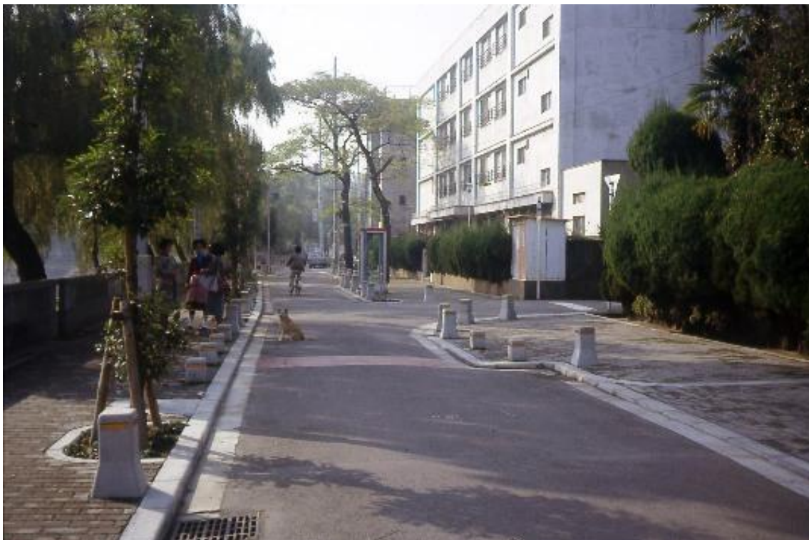
Figure 1 Traffic calming in "Yuzuriha Road" in Osaka's Nagaike-cho (Source: https://ja.wikipedia.org/wiki/コミュニティ道路 )
