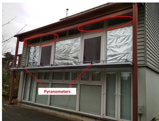
Figure 4: External view of the south façade of the dwelling with the location of the pyranometers. Most glazed areas were covered to minimise the effect of solar radiation.
