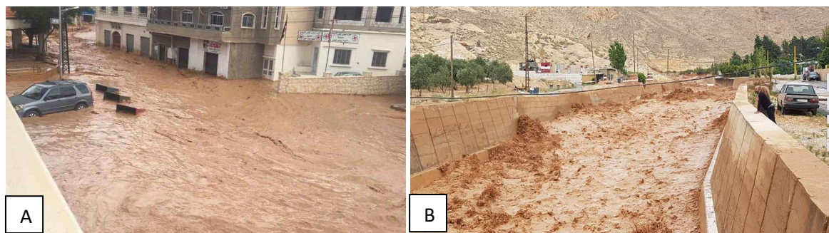
Photo 3.- A: The main road crossing the village was submerged and closed for several hours during the mudflow of June, 2018. B: the channel constructed after the sail of 1994 was flooding during the sail of June, 2018
