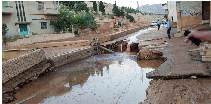
Photo 4.- Roads and buildings affected by the sail of June 2018
