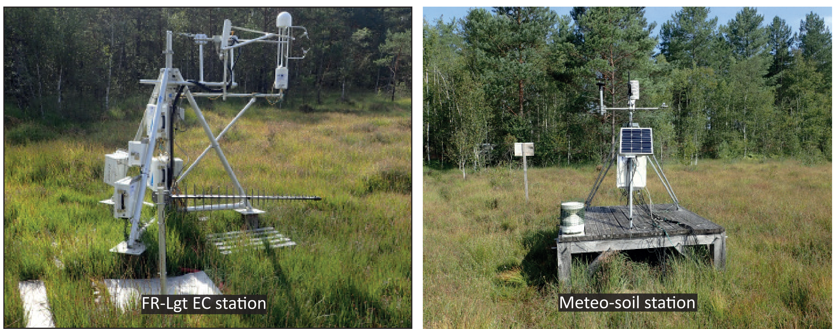
Location of La Guette peatland, and illustrations of the tower and its associated meteo-soil station.
