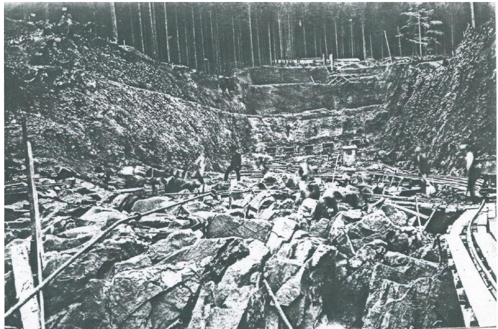
Figure 4. Excavation made in the slope of the Szyndzielnia mountain (the south-eastern part of the dam) during the building of the water dam in Wapienica site [4].
