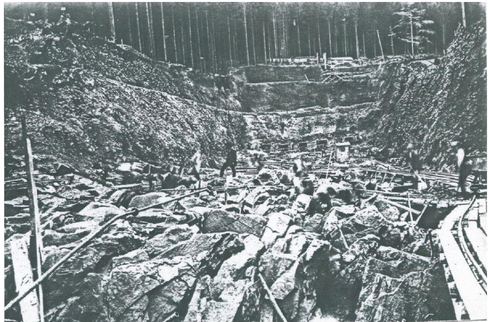
Figure 4. Excavation made in the slope of the Szyndzielnia mountain (the south-eastern part of the dam) during the building of the water dam in Wapienica site [4].
