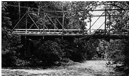
129. Quaker Bridge, across the Croton River in Westchester County, New York.
