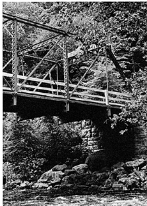
130. The compression members are hollow lattices.
