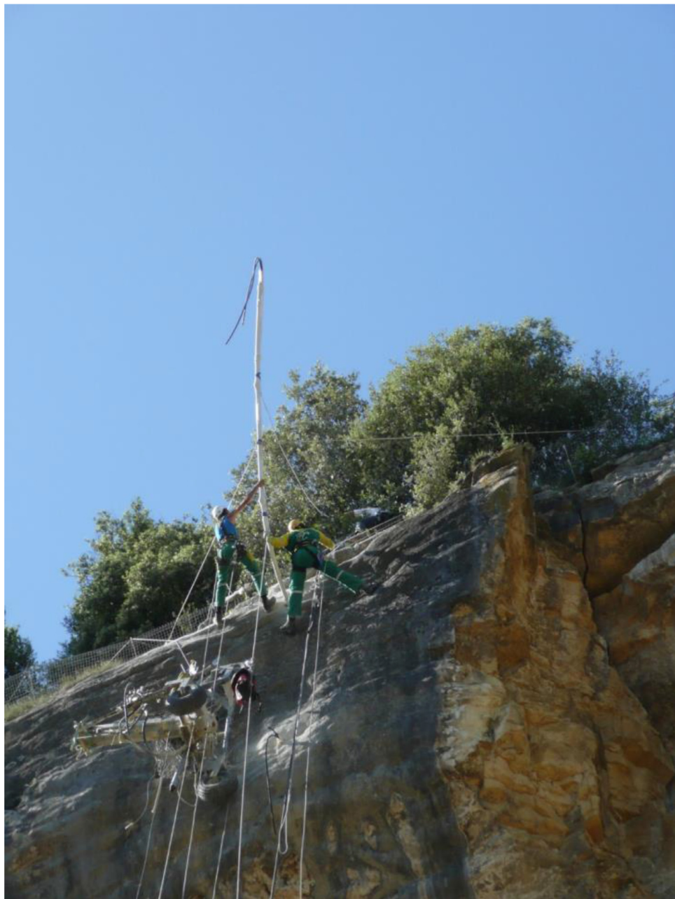
Fig. 1. Installation of borehole extensometer in pre-drilled borehole.
