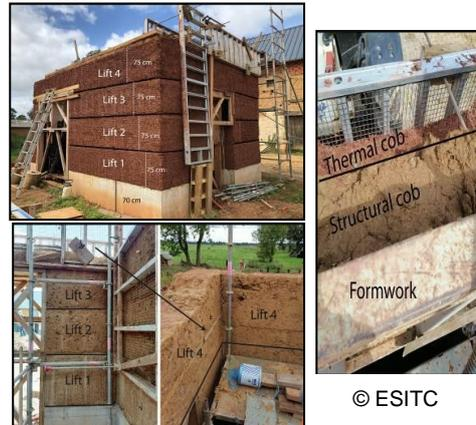
Fig. 1: outdoor and indoor view of the earth-based building
