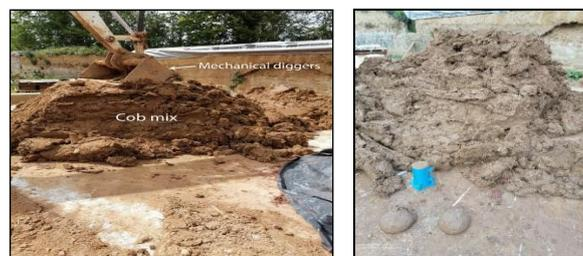
Fig. 6: The cob mixes on the construction site
