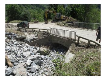
**Figure 2.** Effect of a sediment pulse at a bridge section of the Ruisseau de la Gorge (France), a stream that was known by local engineers as having been inactive for decades. The transported material was much finer ( $D_{50} = 96 \text{ mm}$ ,  $D_{84} = 169 \text{ mm}$ ) than the bed in place ( $D_{50} = 250 \text{ mm}$ ,  $D_{84} = 413 \text{ mm}$ ).
