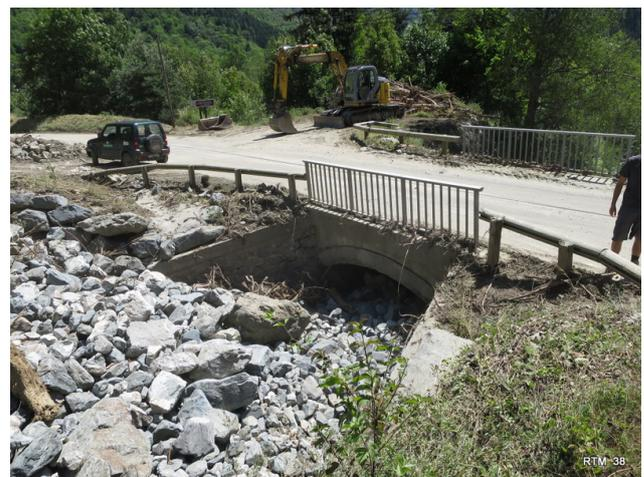
**Figure 2.** Effect of a sediment pulse at a bridge section of the Ruisseau de la Gorge (France), a stream that was known by local engineers as having been inactive for decades. The transported material was much finer ( $D_{50} = 96$  mm,  $D_{84} = 169$  mm) than the bed in place ( $D_{50} = 250$  mm,  $D_{84} = 413$  mm).
