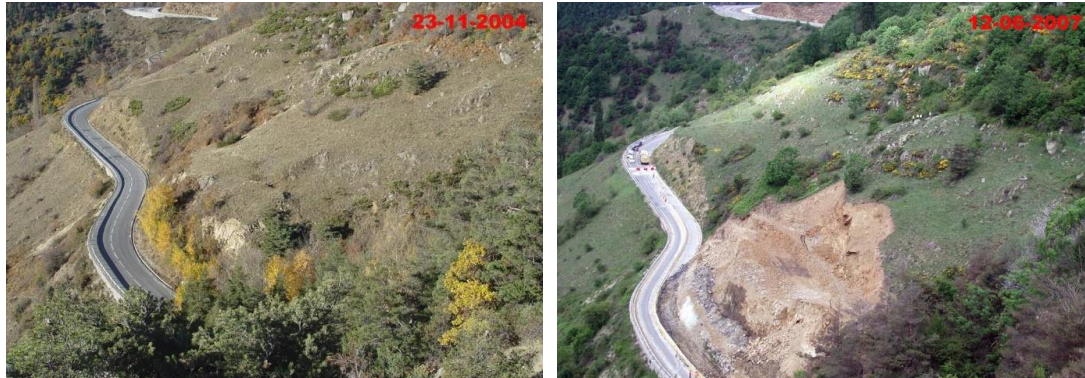
Figure 5. Le Pallat - Sauto slope, before and after 2007 landslide.
