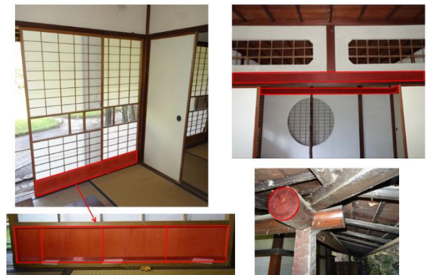
Figure 4: Example of measured timbers (in red). Left: the lower parts of shōji; Top right: tie beams; Bottom right: an outdoor round beam.
